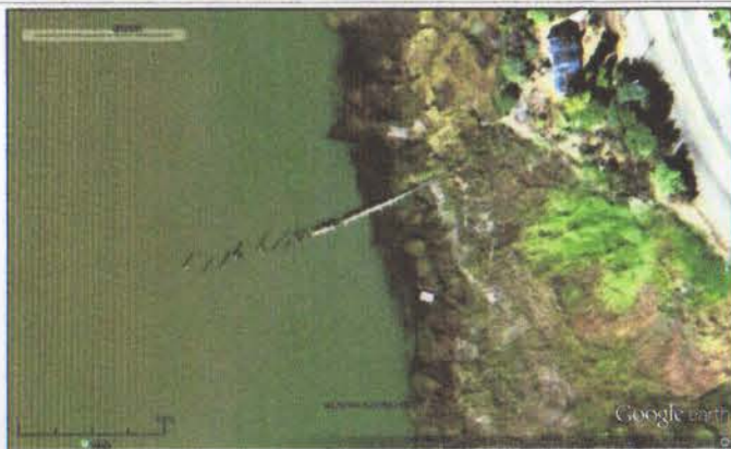
AERIAL PHOTO SHOWING THE EXISTING PIER AND DOCK LOCATION IN 2004.
