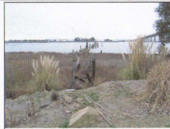
LOOKING WEST FROM THE SHORE, WHERE THE PIER BEGINS
