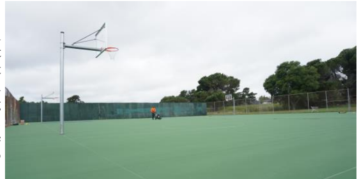
Renovations at Setterquest Park included the addition of two basketball courts and tennis courts resurfacing.
