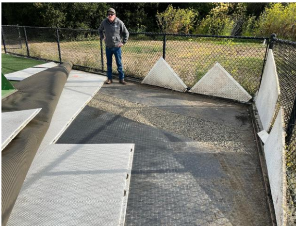
Photo #12 Geofabric and Drain Trench
