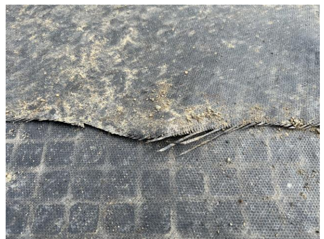
Photo # 13 – Geofabric Close-up
