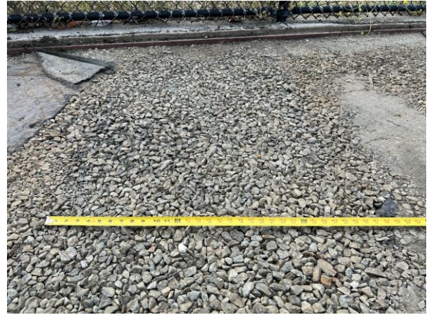
Photo #15 – Infiltration Trench
