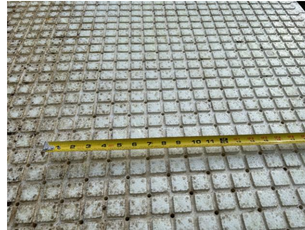
Photo #14 – Bottom side of Underlayment
