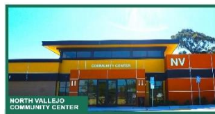
North Vallejo Community Center 1121 Whitney Avenue Vallejo, CA 94589
