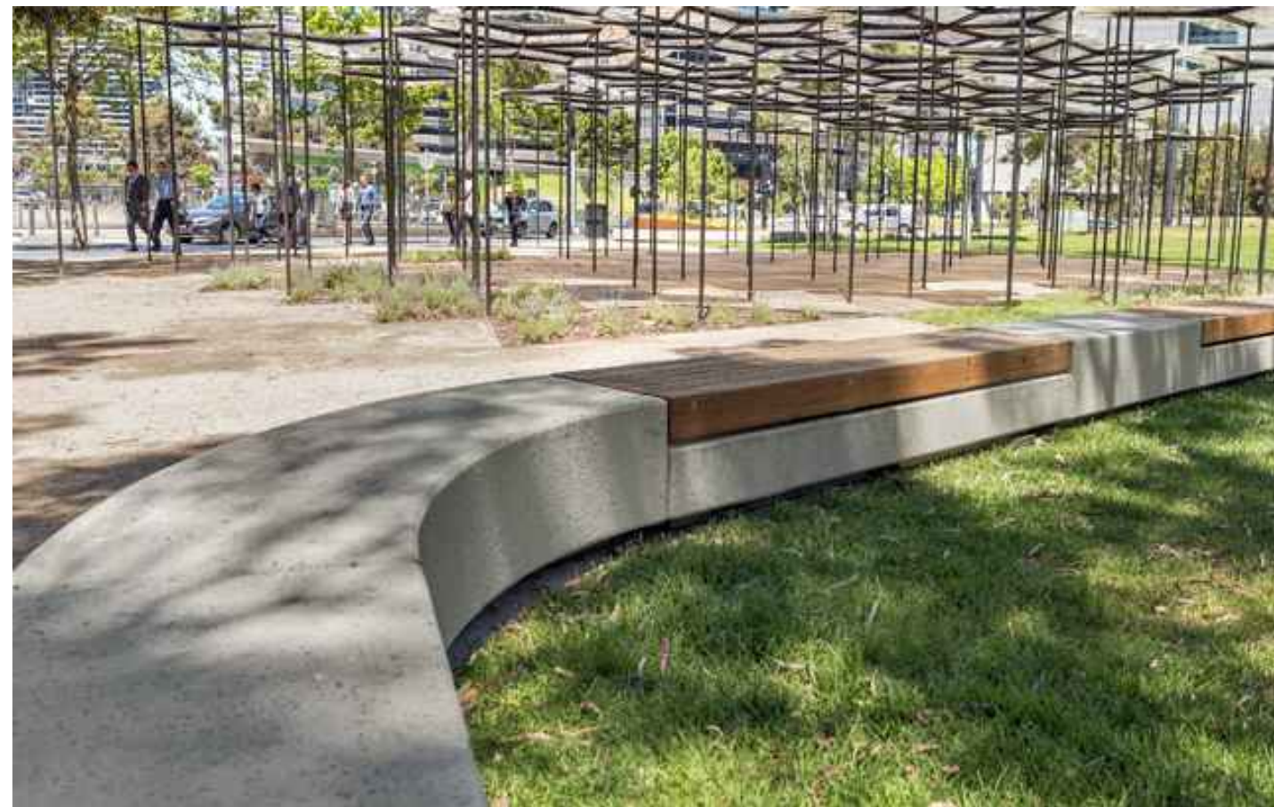
PRE-CAST CONCRETE SEAT WALLS WITH WOODEN BENCHES
